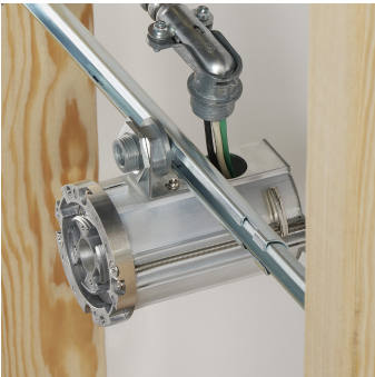
Connect power from conduit to junction box.
