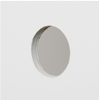
Cut hole in desired location.
