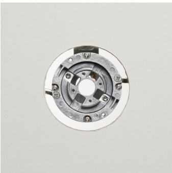
Install the drywall.
